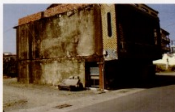
(Fig.2) Due to the soft ground, the original two-floor building has currently sunk to simply one-and-a-half floors.
