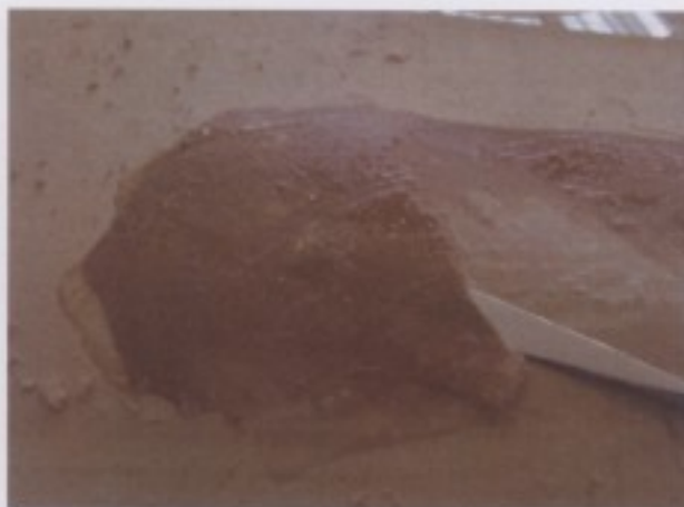
It's easy to take off the backing paper by piloting the 3% MC with water. (wait for 15minutes)
