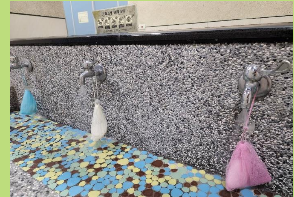
廁所洗手台加裝省水裝置
